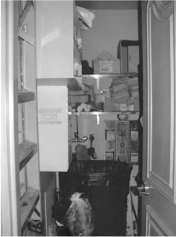
Figure 11-11 A typical public area utility closet at the Bellagio. Note the chemical mixing station at the rear of the closet. (Photo courtesy of Bellagio, Las Vegas, an MGM Mirage property.)
